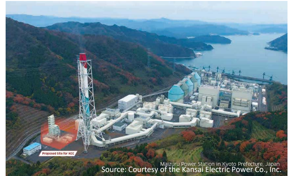
CCS Demonstration Plant at Maizuru Power Station
